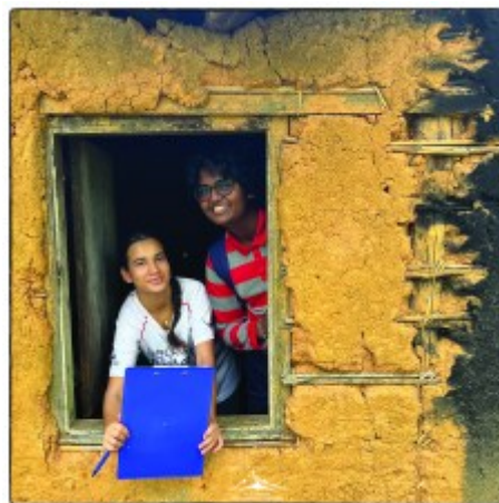
Maya and Chirath explore a disused traditional adobe home. Most houses are now made of concrete bricks with asbestos roofs.
